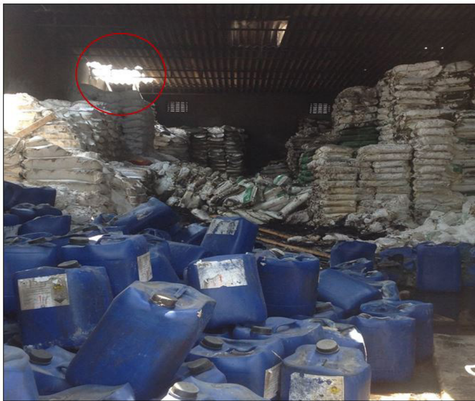
Figure 3: An overview of the fire effected warehouse showing the blown off roof over the area where maleic anhydride was stored indicating a low intensity explosion.
