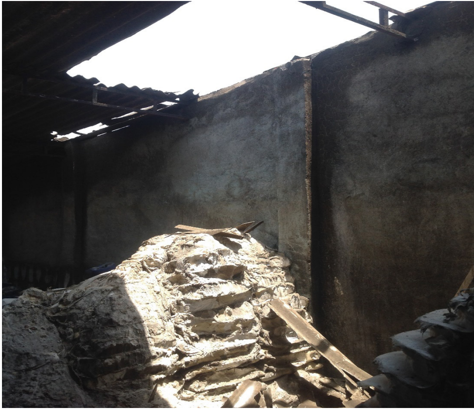
Figure 5: A view of fused Sodium Sulphate bags. The blown off roof due to low intensity explosion can also be seen in the figure
